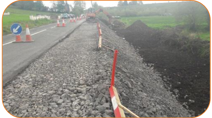
Verge Strengthening works at Gleann on R284 funded by Specific Improvement Grant
