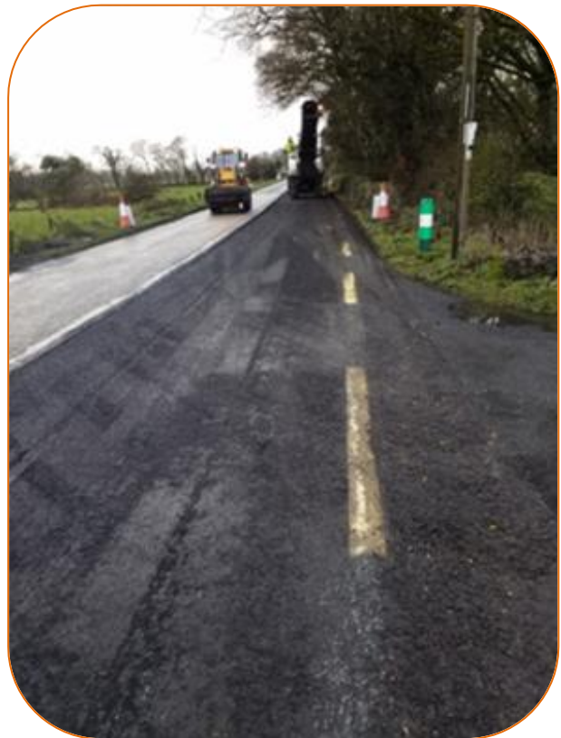
N17 Tobertelly pavement strengthening
