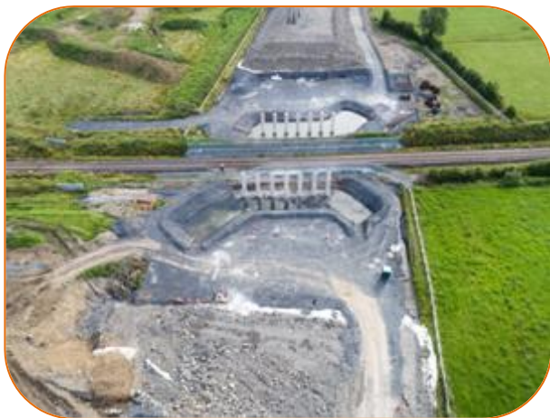
September 2019 – Railway Bridge Works at Maugheraboy
