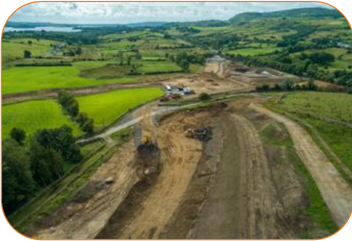
Looking south toward the tie-in south east of Castlebaldwin
