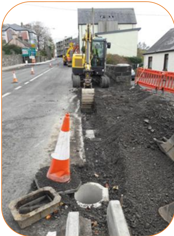
Footpath, drainage and road pavement works N59 Ballysadare
