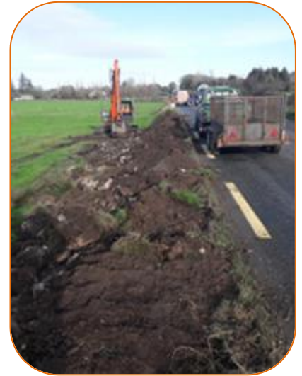
Sight line improvements on N17 at Tobertelly
