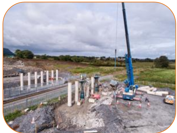
Construction of rail bridge over Dublin to Sligo Line
