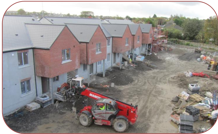
View towards Block B: Knappagh Beg Court, Knappagh Road
