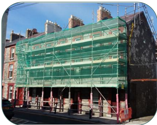
Conservation works underway to 79-81 John Street, Sligo – funded under the Built Heritage Investment Scheme 2019
