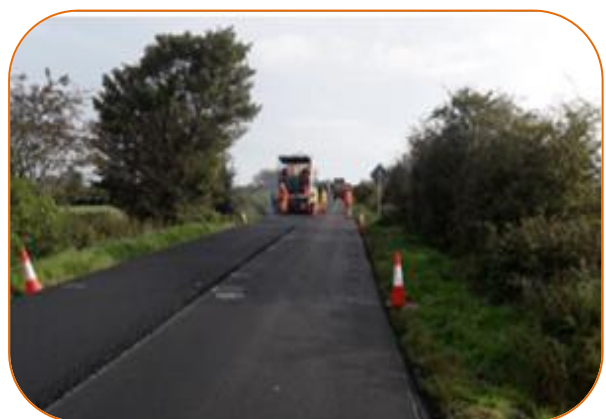
Pavement Strengthening at N59 Rathglass
