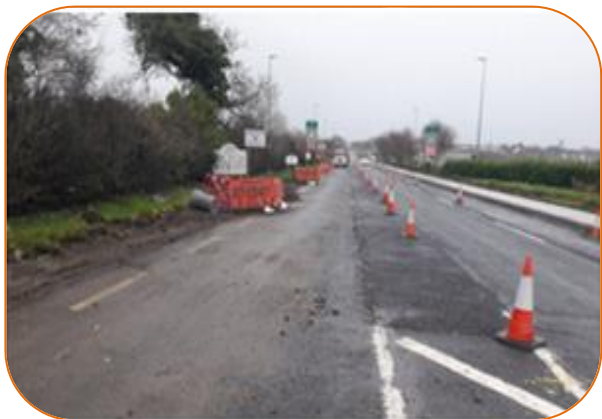
Footpath, drainage, road reconstruction and strengthening works at N15 Shannon Eighter
