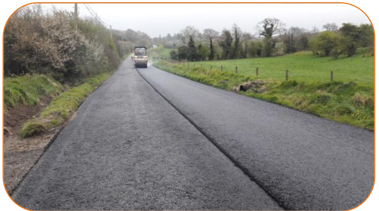
Road Strengthening Works Ballymote area funded under Restoration Improvement Grant
