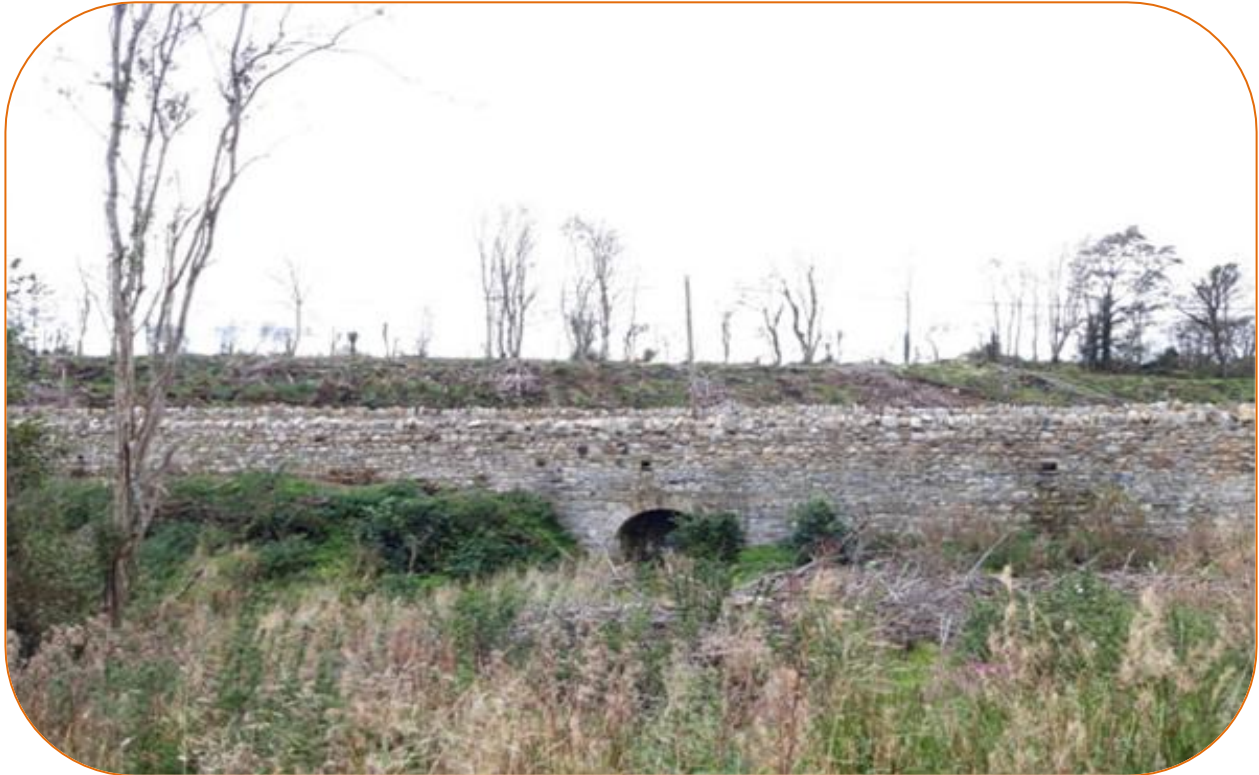
Srarevagh Bridge north of Lissadell completed in July 2019
